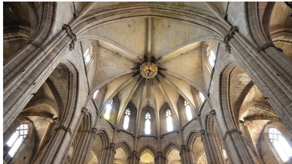
Figure 15. The main keystone of the apse of the Tortosa Cathedral (1346–1441). Image by the authors.
