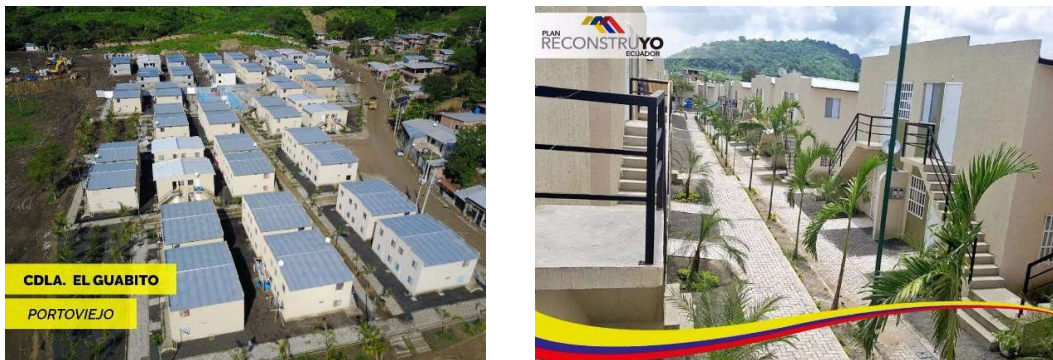
Figure 14 (a, b). “ El Guabito ” Public Housing Project.
