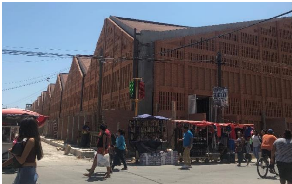
Fig. 3. City market’s damages after the disaster in September 2017 vs. City market under reconstruction. Image: Local community member.
