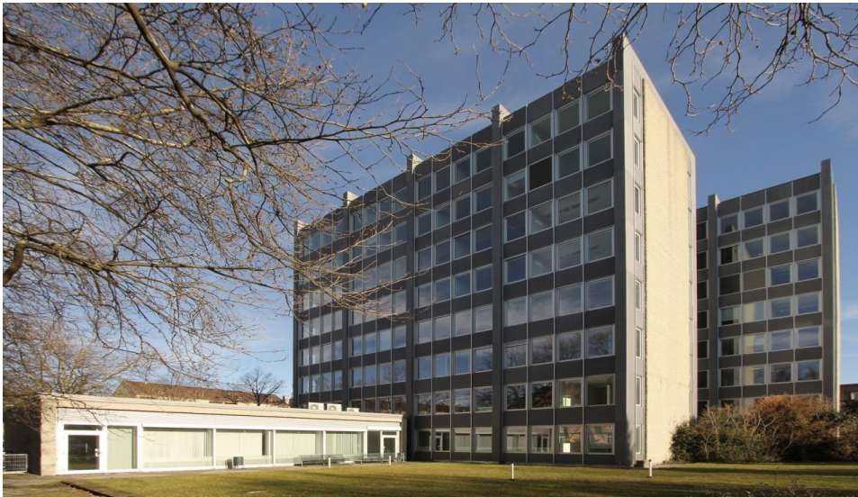
Figure 24. View of the building exterior.
