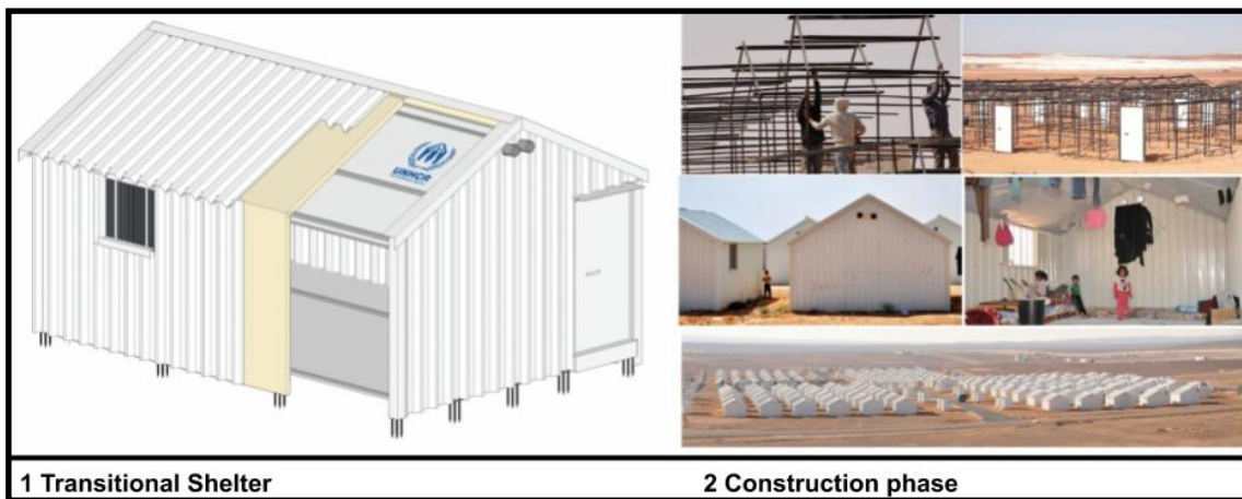
Figure 4.54 (1) T-Shelter Design (2) Collective Images Of Construction Phase And T-Shelter Indoor Space. Edited by the author, 2020. Adapted from T-Shelter for Azraq Refugee Camp, by UNHCR, (2015_c). Copyright 2015 by UNHCR
