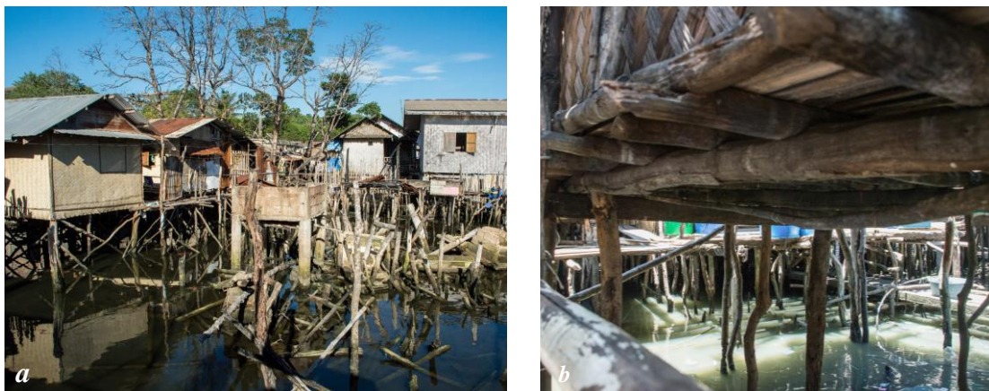
Figure 11a. Coastal settlement of Barangay 1, Figure 11b. Example of typical timber post built directly in the water. Source: Pictures by Erika Palmieri
