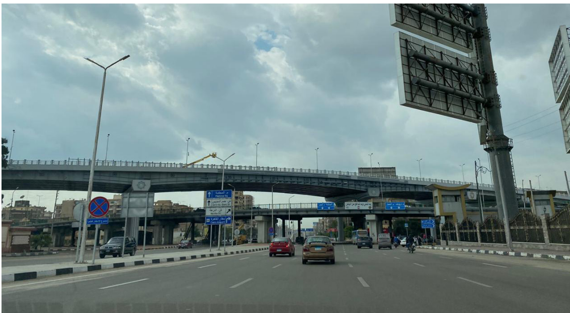
Figure 12 shows a recent photograph of one of the modified areas; road changes and a bridge constructed above a pre-existing one. Source: Samaha, O, (2020).
