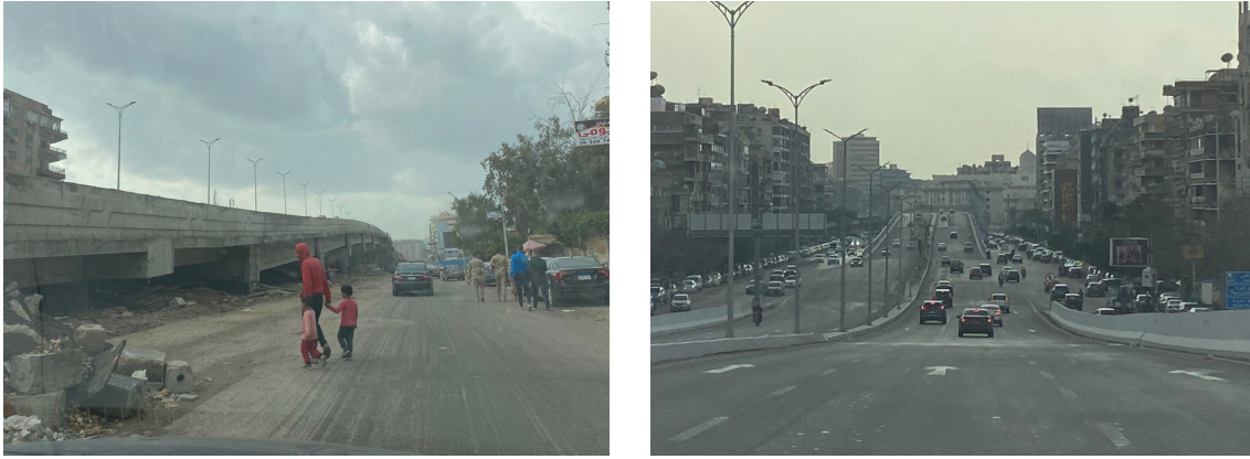
Figure 19 left shows the experience of walking in Heliopolis during road changes and bridge construction. Source: Samaha, O. (2020). Right shows a bridge constructed right after pre-existing bridge in El-Sayed El-Merghany street. Source: Samaha, O. (2020).
