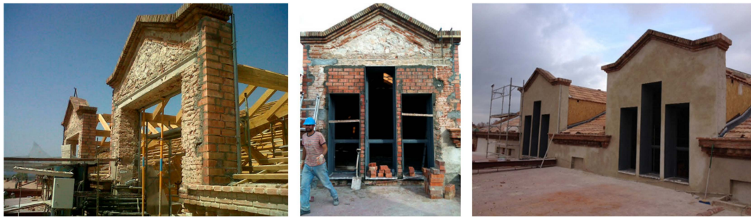
Figure 30. Dormer windows of the production nave during restoration ( left and center ). Dormer windows of the production nave after restoration ( right ).
