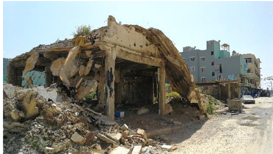
Figure 31. Houses in ruins: the living memory of the 2007 war Source: Author's archive.
