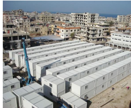
Figure 7. Deployment of temporary shelters Source: www.platform-ad.com/cold-river-reconstruction-of-nahr-el-bared-refugee-camp-by-unrwa-nbrc/
