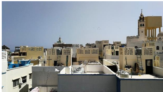
Figure 18. Perforated concrete blocks with “arabesque” patterns used in the new buildings
