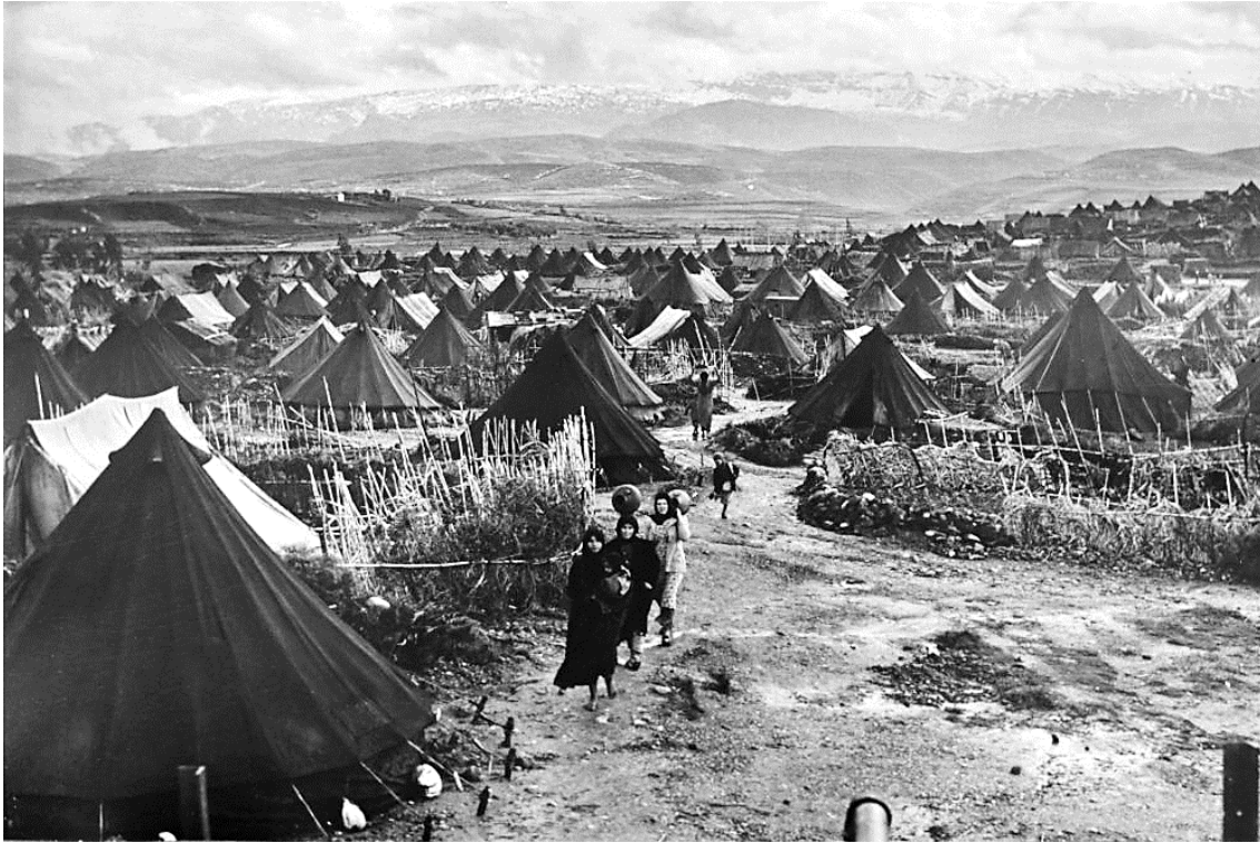
Figure 4. Nahr el-Bared Refugee Camp when deployed as an emergency response.
